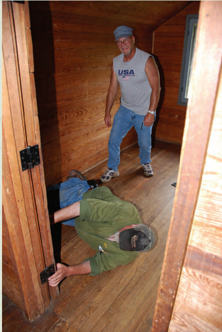
Gary Johnson & John Cummins (standing) replacing missing hardware with ones they recreated.
